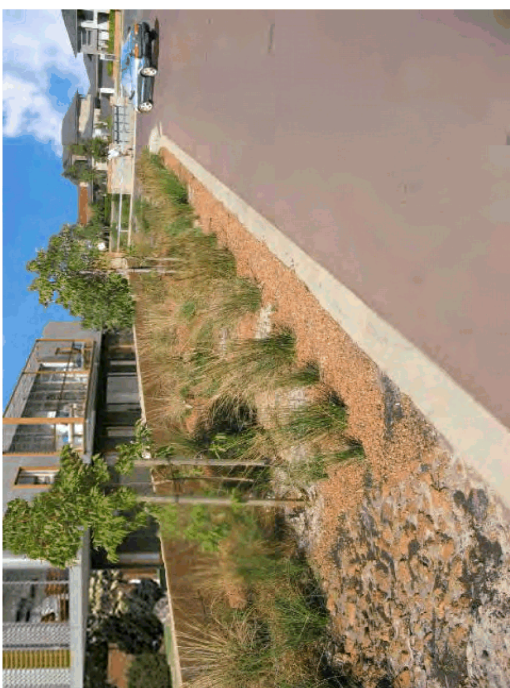
PHOTO EXAMPLE OF VERGE PLANTED BIO FILTRATION
