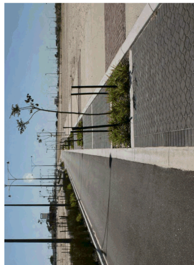
PHOTO EXAMPLE OF TYPICAL BRICK PAVING WITH BIO FILTRATION POCKETS OR RAINGARDEN
