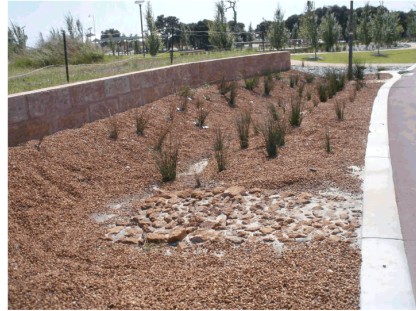
PHOTO OF - TYPICAL VERGE SWALE
