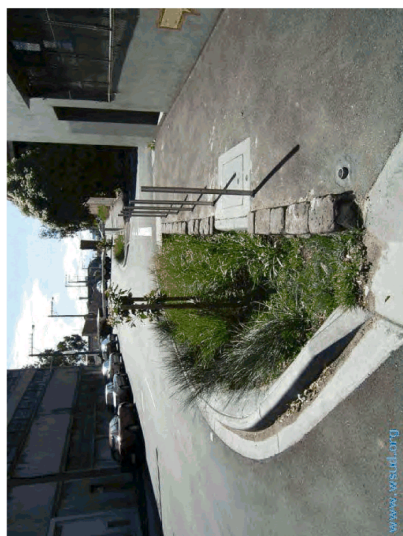
PHOTO EXAMPLE OF BIO FILTRATION POCKET FOR RAINGARDEN WITH SIDE ENTRY PIT
