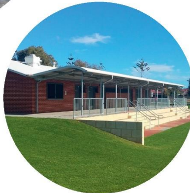
Sports upgrade One of three new amenities buildings constructed during the year, Belhaven Park has new unisex changing rooms, a fully fitted kiosk and servery, time-locked public toilets, store rooms, and first aid and umpires rooms. A covered veranda and terraced seating complete the picture.
