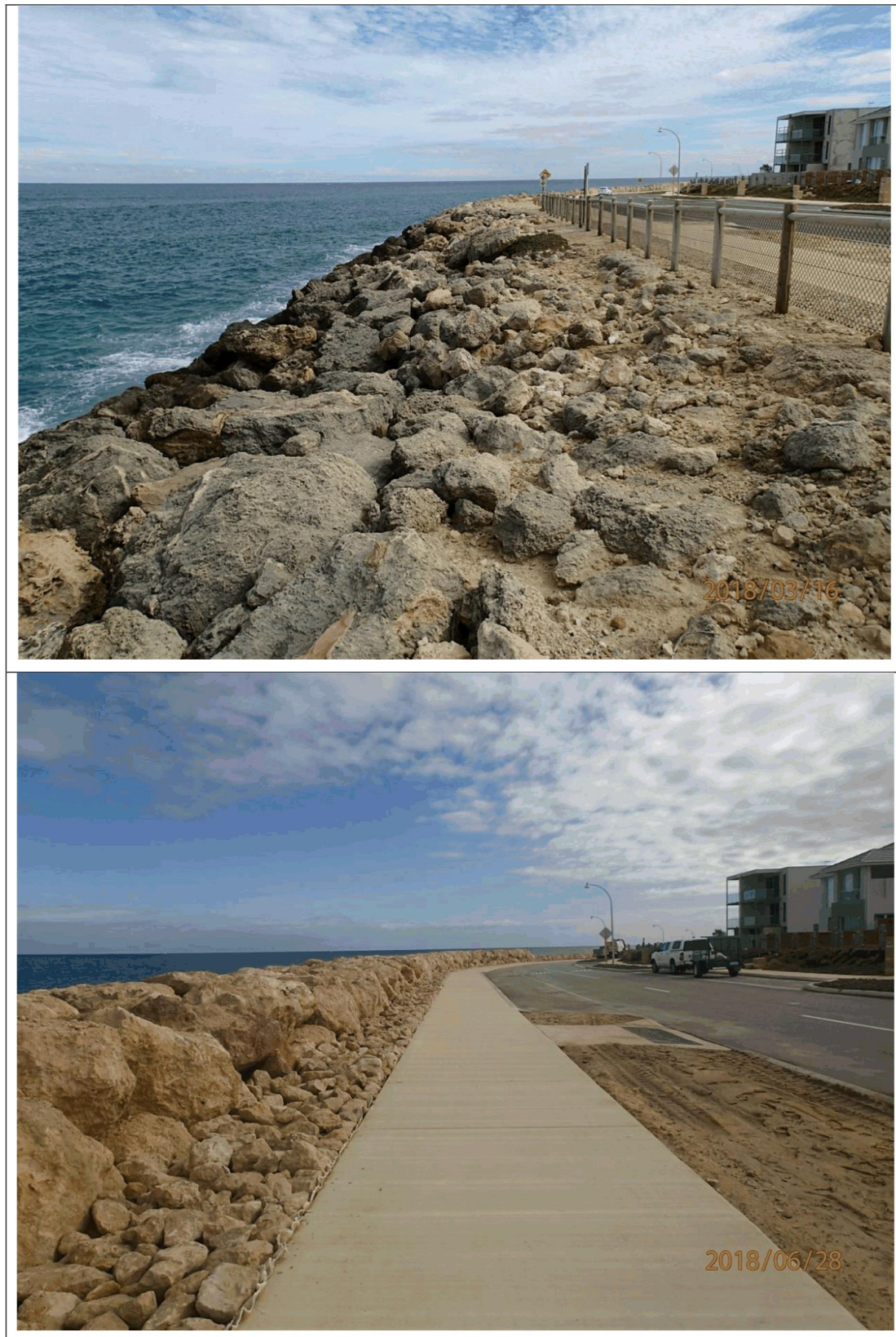
Figure 3. Phase 1 Maintenance Works - Pre Construction (top) and Post Construction (bottom)
