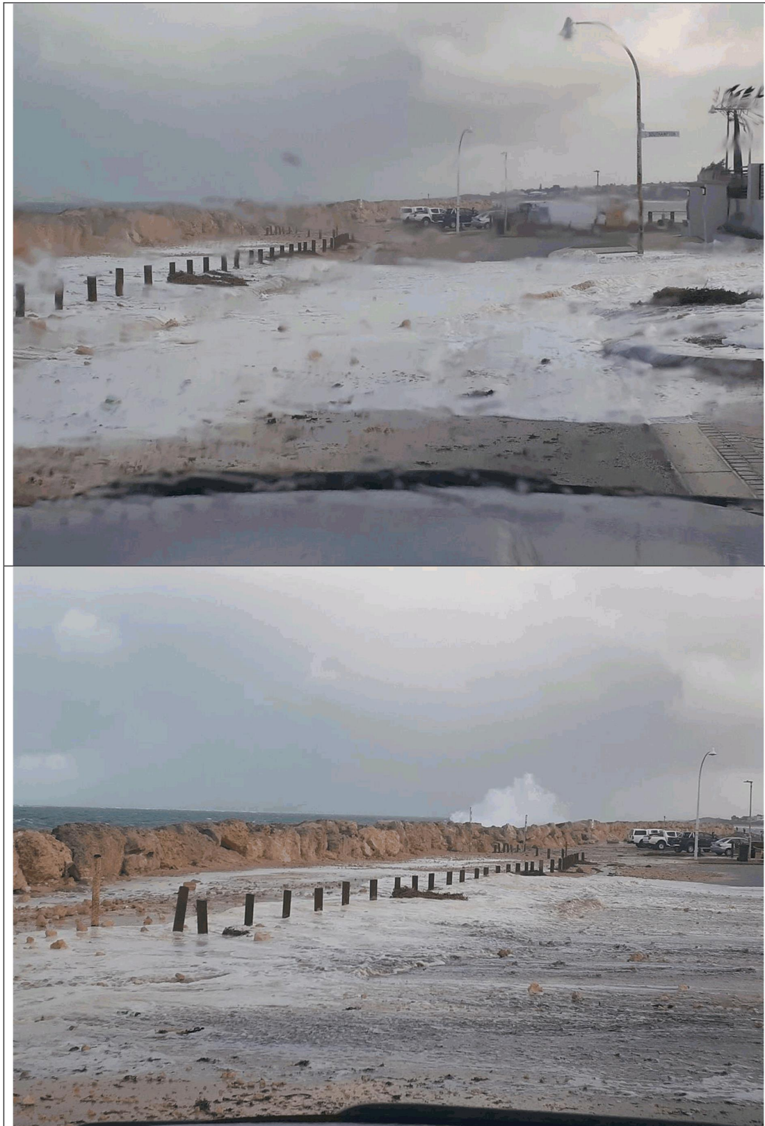
Figure 6. Wave overtopping at Segment 4.
