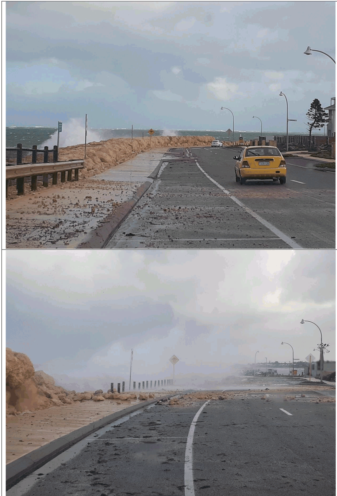
Figure 5. Segment 3 after maintenance works with no rock debris and minimal wave overtopping (top), Segment 4 with excessive wave overtopping and rock debris displaced onto the path and road (bottom).
