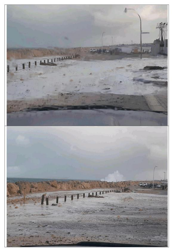
Figure 6. Wave overtopping at Segment 4.
