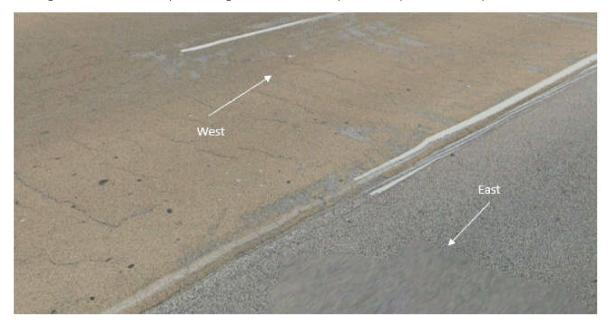
Figure 3-2: Westbound approach lanes onto Wanneroo Road showing delamination and crescent-shaped cracking (Image captured March 2020)
