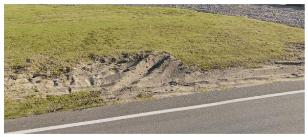
Figure 3-7: Typical Sand subgrade (SLK 0.900)
