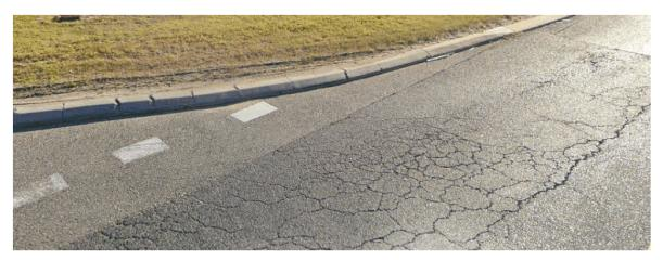
Figure 3-5: Pavement failure at Rigali Way slip road exit (Image captured October 2019)
