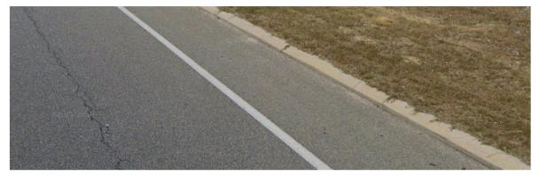
Figure 3-6 - Longitudinal cracking evident between SLK 1.35 to Hartman Drive (Image captured March 2020) The table below summarises the pavement condition from Wanneroo Road to Hartman Drive. Table 3-4: Wanneroo Road to Hartman Drive Visual Condition Assessment Summary
