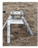
Concrete-less pile footings to minimise ground disturbance
