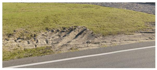
Figure 3-7: Typical Sand subgrade (SLK 0.900)
