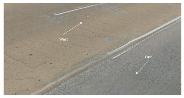
Figure 3-2: Westbound approach lanes onto Wanneroo Road showing delamination and crescent-shaped cracking (Image captured March 2020)
