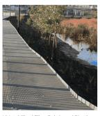
UV stabilised Fibre Reinforced Plastic (FRP) grating and kick-rails to be used for the bird hide boardwalk
