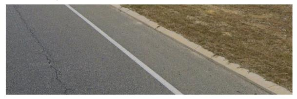
Figure 3-6 - Longitudinal cracking evident between SLK 1.35 to Hartman Drive (Image captured March 2020)
