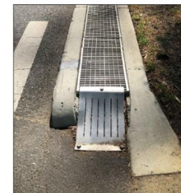
DETAIL-1 (STRIP DRAIN) NTS
