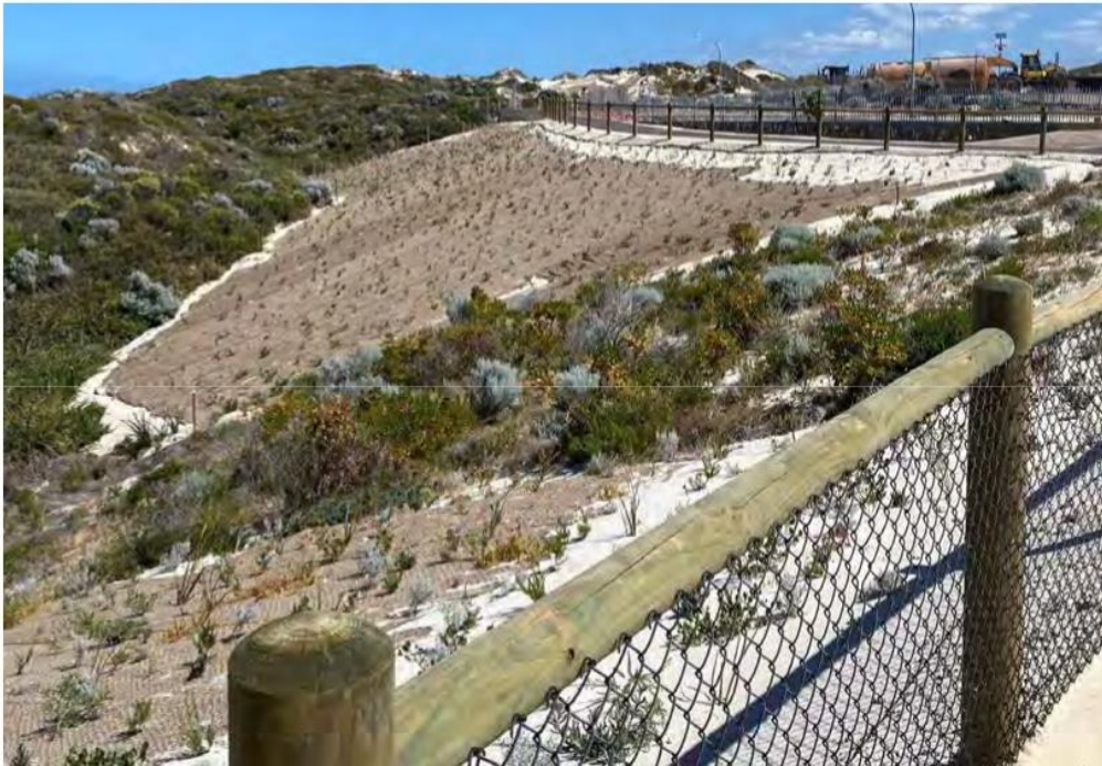
Plate 1: Example of Coir matting used in coastal dunes with tubestock installed.
